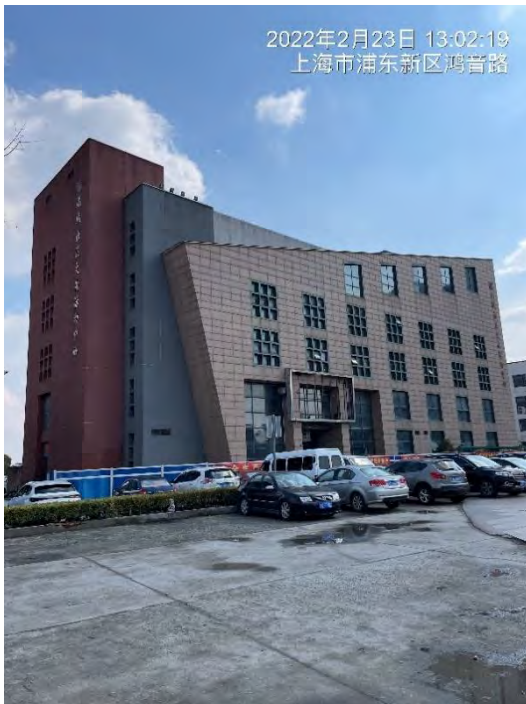
Photo 1: Entire building (under refurbishment)
